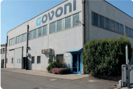
PRODUCTION PLANT 1 Crevalcore, Italia
